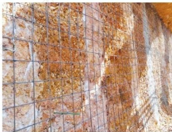
桩间挂网喷浆
